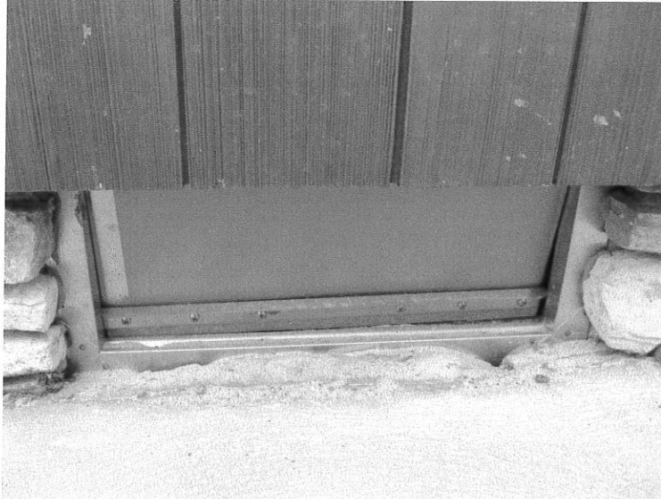
Vents (6) USA Vents Certified for 250 S.F. Each Date Taken:05/29/2009
