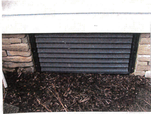
CRAWL SPACE DOOR SYSTEM VENT - TYPICAL OF 4
