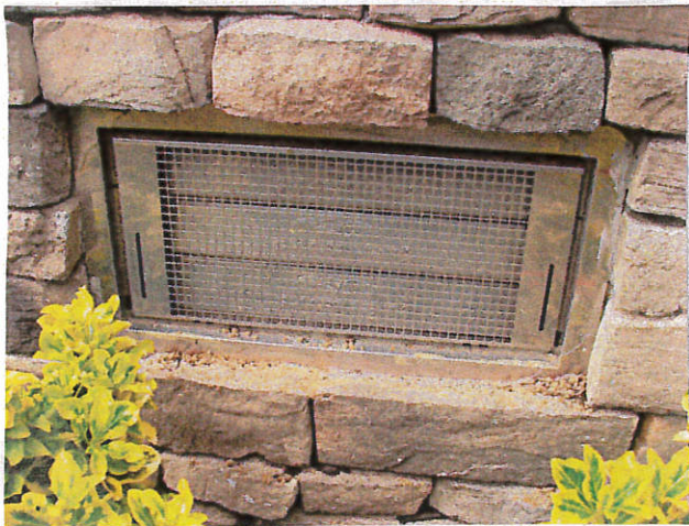
SMART VENT - TYPICAL OF 2
