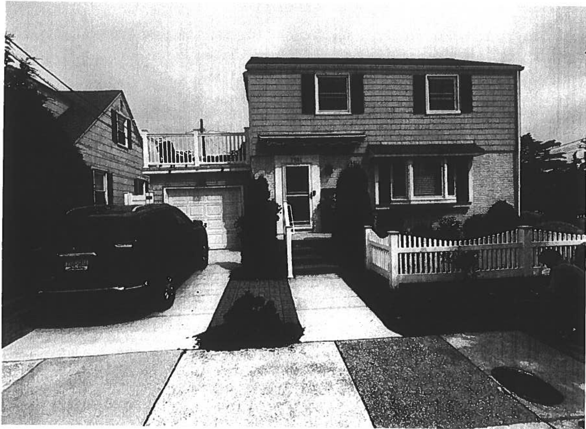
FRONT VIEW OVERALL
