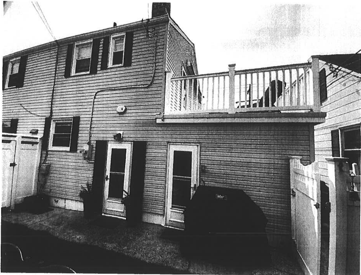
REAR VIEW GARAGE
