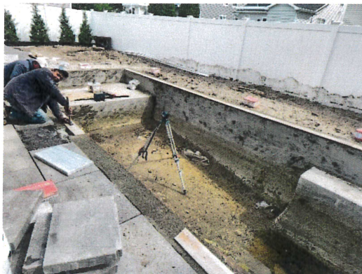
Grading is towards the neighbor – need swale or timber ties. Pool is incomplete
