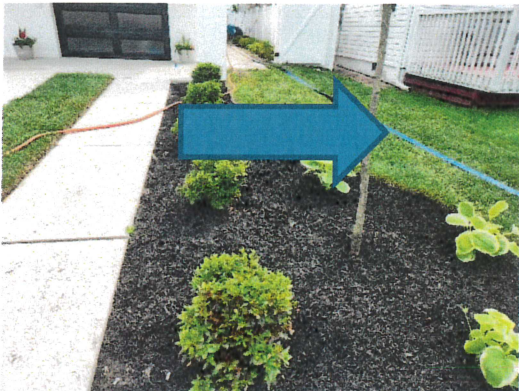
Grading is towards the neighbor – need swale or timber ties. Pool is incomplete
