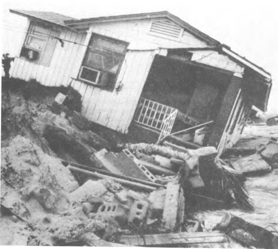
Flood water velocity produces lateral forces that can cause scour and result in collapse of foundations (above left), increase the magnitude of debris impact loads (below left), and dislocate buildings from their foundations (below).
