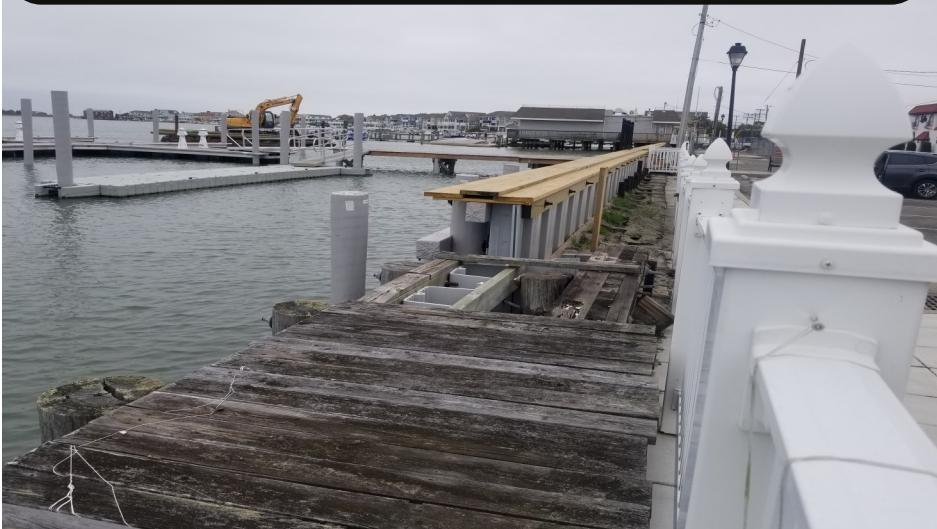
An old section of Bulkhead meets the newly installed section along Amherst Ave.
