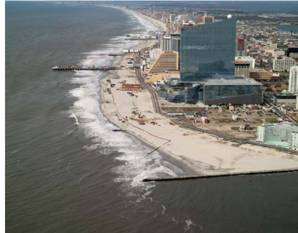
The U.S. Army Corps of Engineers Philadelphia District pumps sand onto the northern end of Atlantic City in 2012 as part of the first full scale renourishment of the project.
